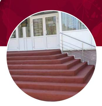
Since 2016, the company has been engaged in tire disposal as well as the production of safety non skid coatings from rubber and EPDM chips, which are used for the improvement of outdoor public facilities (children's and sports grounds), ramps, entranceways, etc. The productivity of its equipment for tire disposal is 1 thousand tons per year, and its productivity totals 30 thous. sq. m of rubber tile per year.
